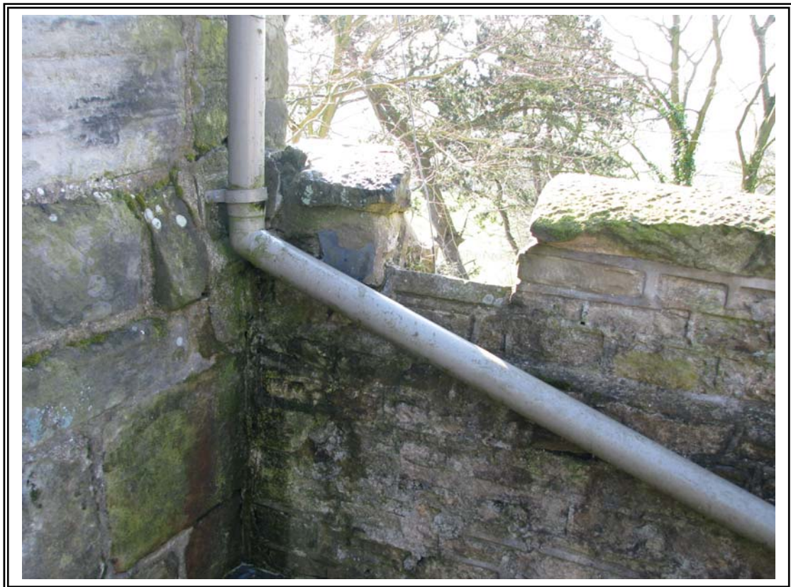
4. Leaking rainwater pipes.
