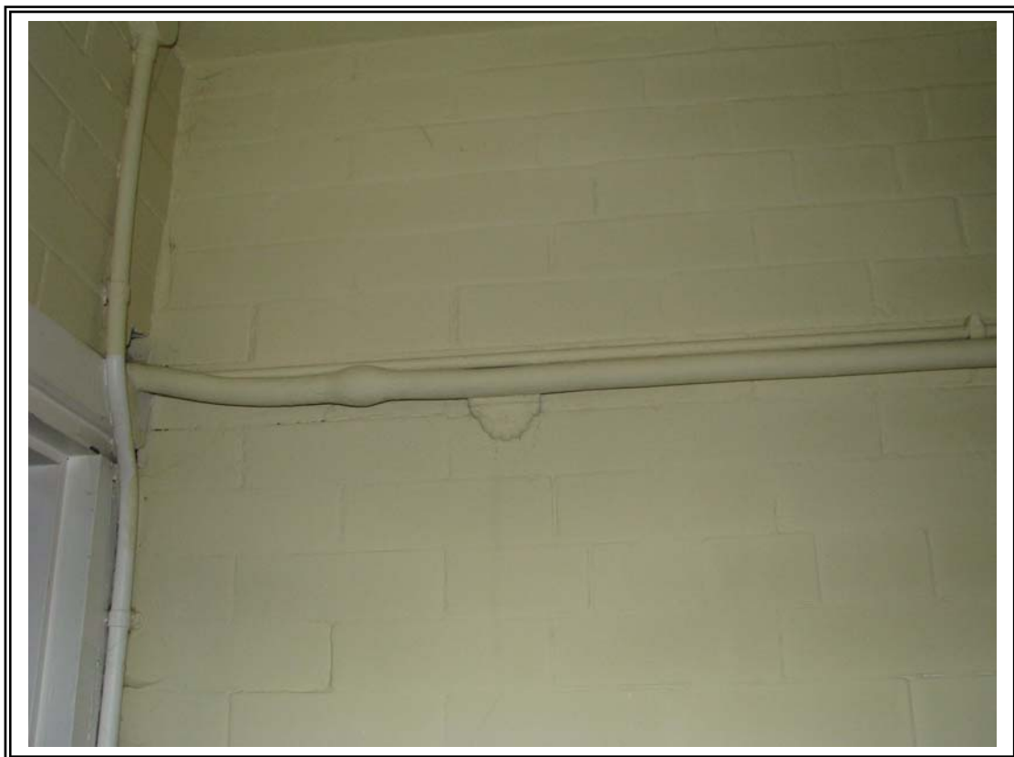
18. Lead pipework.
