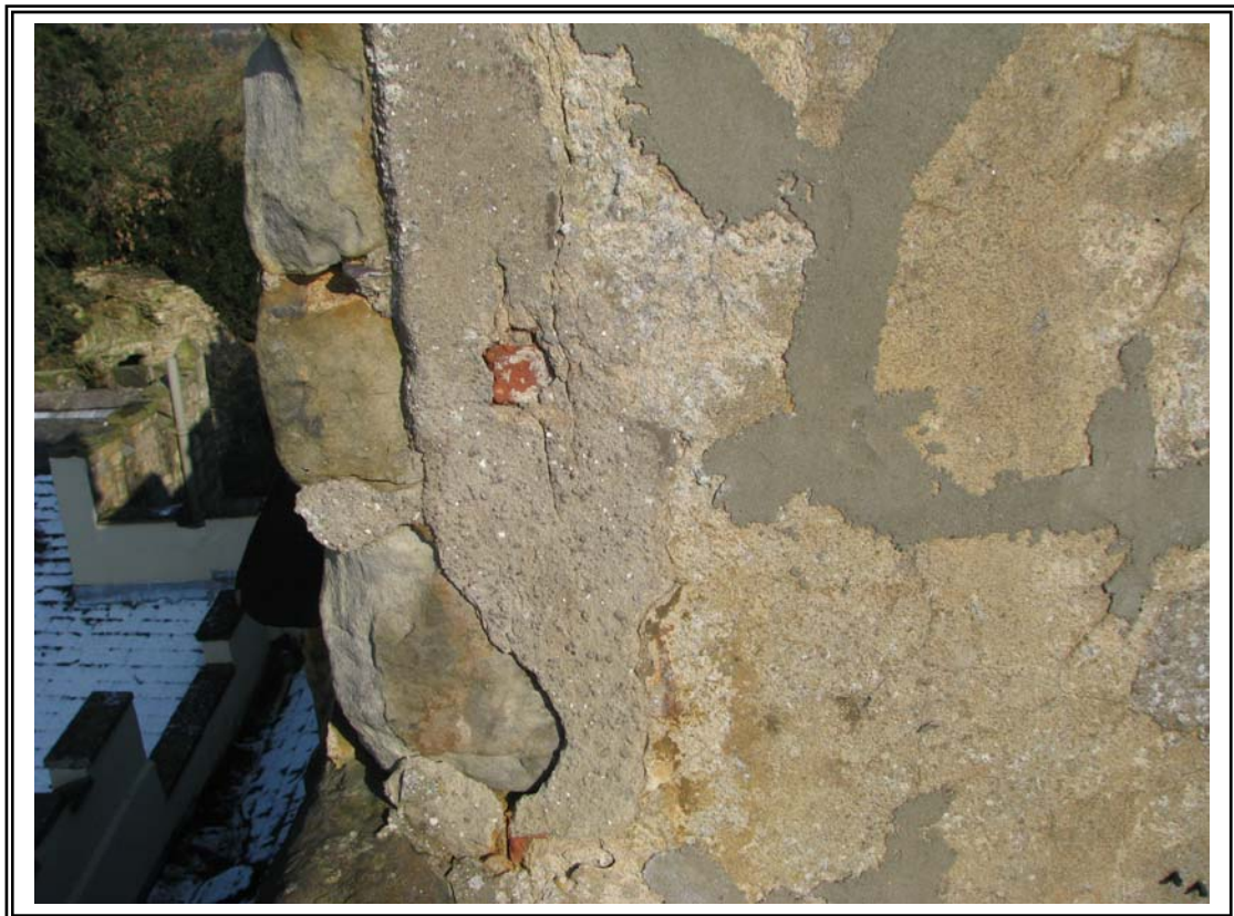
10. Remedial cement mortar pointing.
