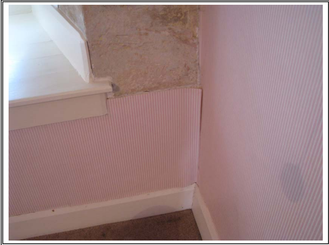
15. Evidence of condensation.
