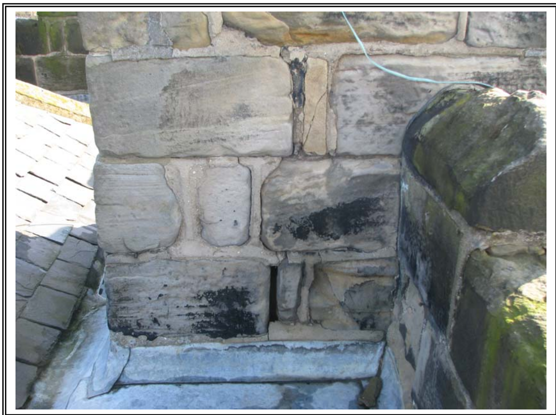
12. Eroded mortar to chimney.
