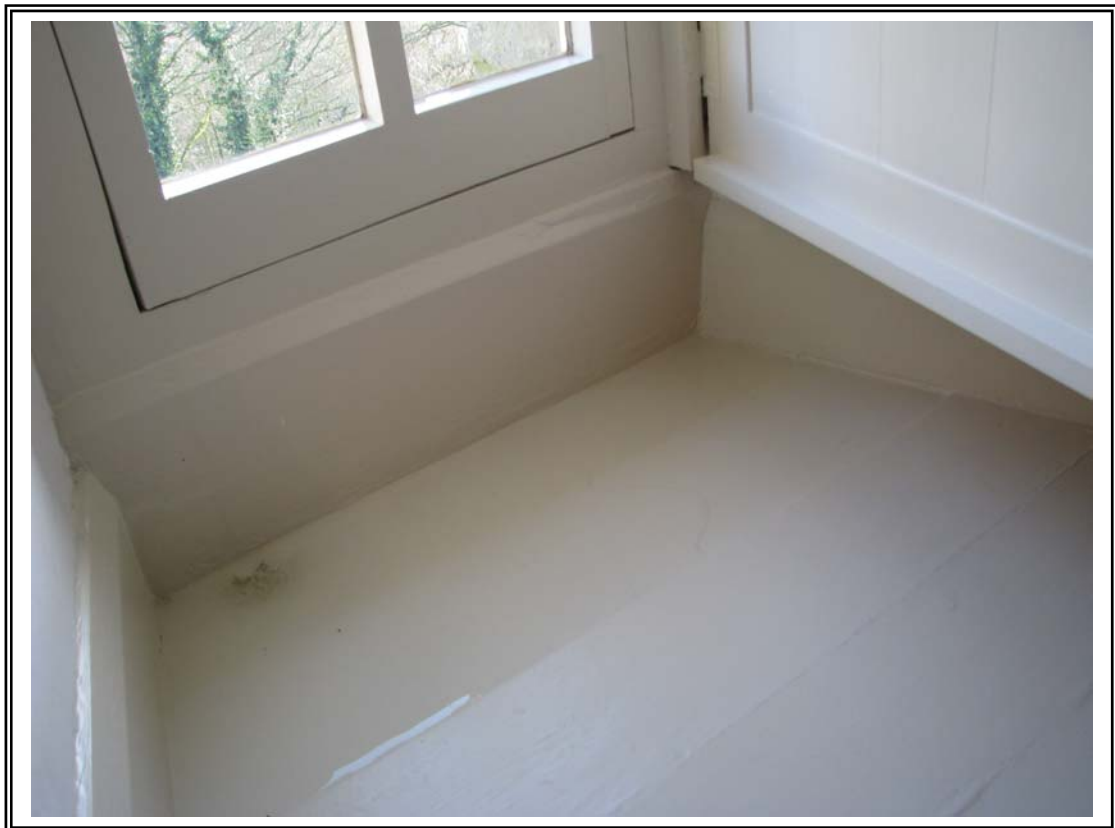
16. Evidence of condensation.
